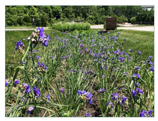
Ohio Spiderwort within the native forb bioretention cell. The monitoring station is in the brown box in the background.
